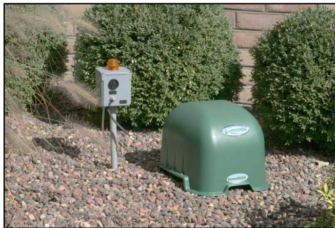
Figure 39, Aero-Alert Installed
