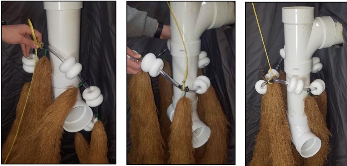
Figure 20, Bio-Brush Cluster installed around Outlet Baffle
