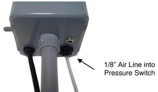
Figure 31, Underside of Alarm
